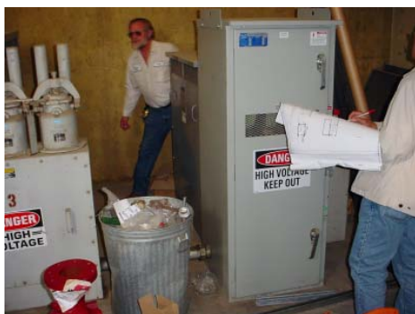
Figure 11 – Indoor service equipment.
