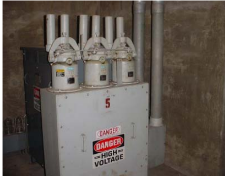
Figure 1 – Oil-filled fuse cut-outs for T-5
