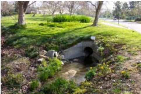
Figure 3 - Concrete headwall discharging site storm drain to open channel located along the northerly side of Campus Drive.
