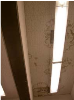
Water damage at ceiling
