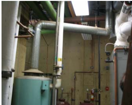
Gas water heater flue
