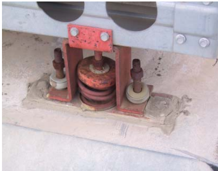
Figure 1 – Example of vibration isolators that are shot and need to be replaced.
