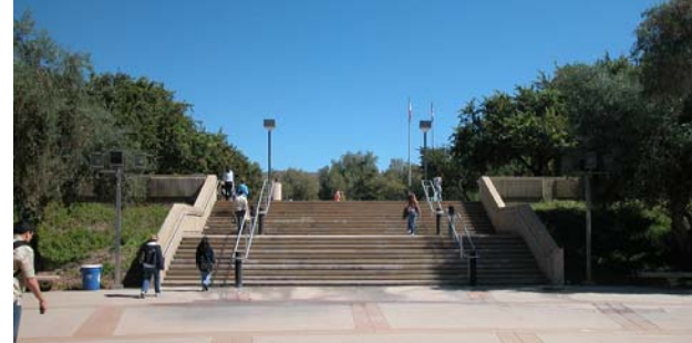
THRESHOLD - STAIR FROM PERFORMING ARTS CENTER
