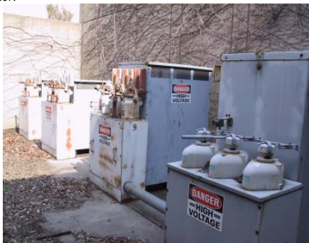
Figure 4 – Main service equipment.
