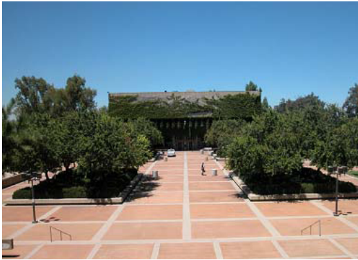
COLORED CONCRETE GRID PATTERN AT HISTORIC CORE OF CRAFTON HILLS COLLEGE
