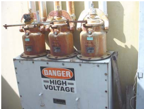
Figure 10 – Oil-filled fuse cut-outs.
