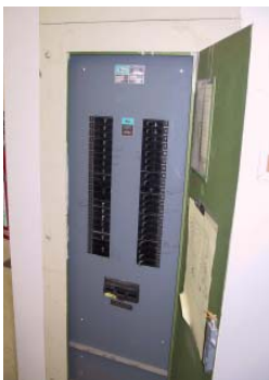
Figure 4 – Zinsco panel board
