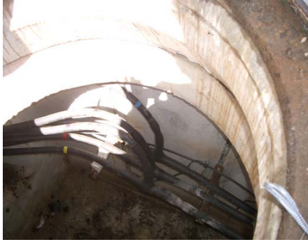
Figure 1 – Electrical manhole.
