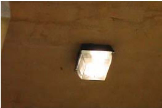
Figure 3.2 – Metal halide – this is a moderate to good color rendering source.
