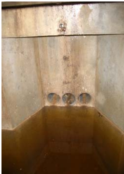
Figure 3 – Available knock-outs. Manhole half-filled with water.
