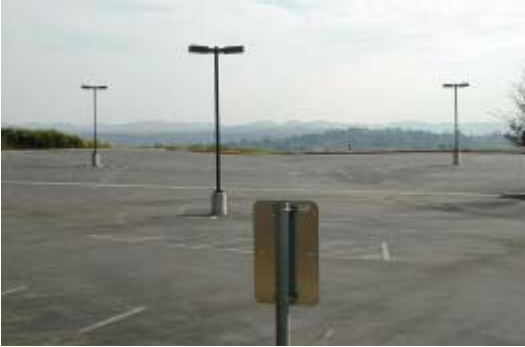
Figure 1.2 – Child Development parking – Low, sparse fixtures inadequate for area of parking lot.
