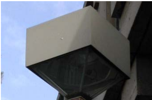
Figure 8.3 – Cut-off optics – Light is directed only below horizontal
