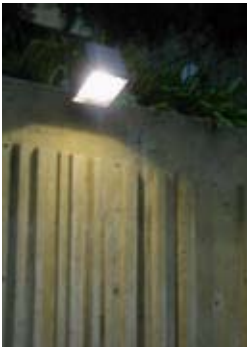
Figure 5.4 – Glare from floodlights actually counteracts the illumination they provide.
