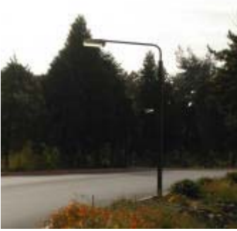
Figure 1.1 – Street lighting - restricted height and wide spacing lead to uneven lighting.
