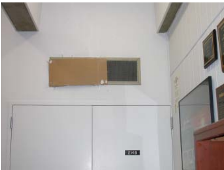
Supply air register - Occupants have partially blocked register as a means of controlling air flow.
