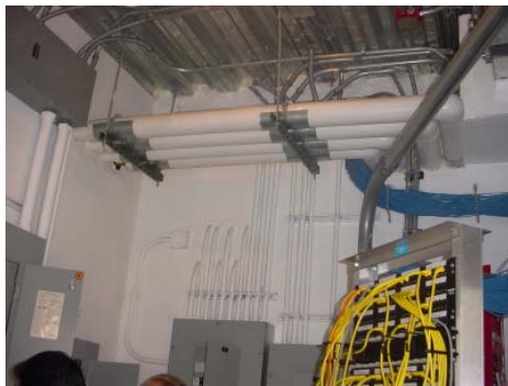
Figure 12 – HVAC pipes above electrical panel.
