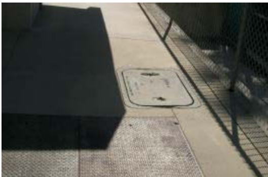
Figure 2 – Pull box at Gymnasium location. Communications cabling is routed through Electrical vault.
