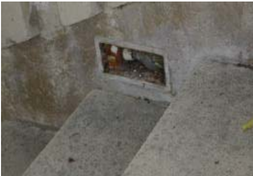
Figure 5.3 – Steplights with polycarbonate lenses will eventually fall to vandalism.
