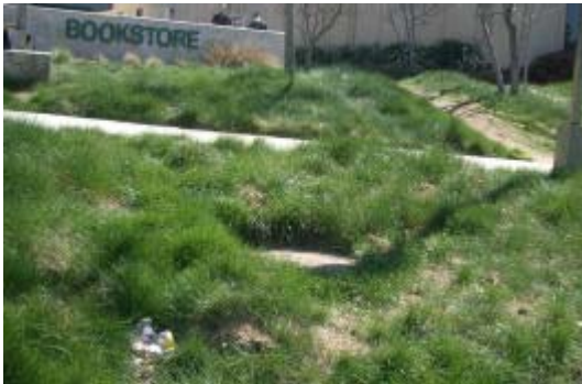
Figure 2 – Manhole location at bookstore is the southern end of campus communications infrastructure spine.
