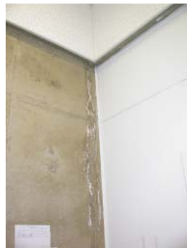
Water damage at wall
