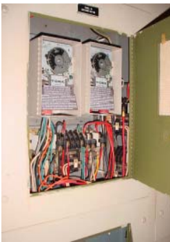
Figure 2 – Panel with time clock
